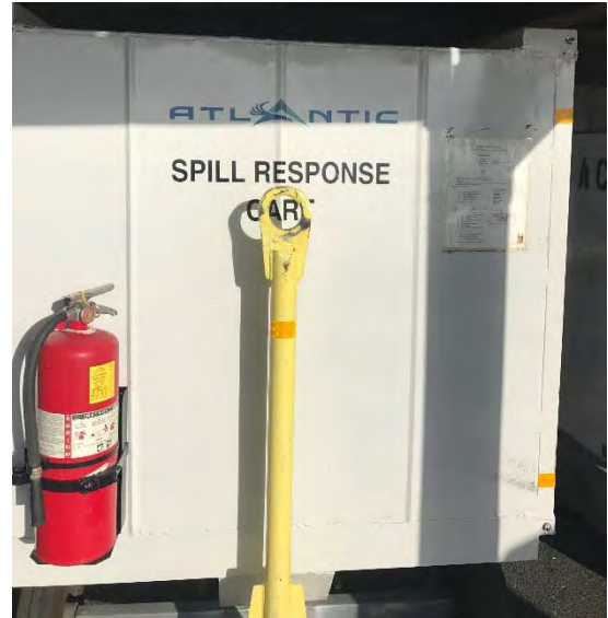
Example of a mobile spill response cart which includes a spill response plan and is stocked with appropriate spill cleanup materials.
