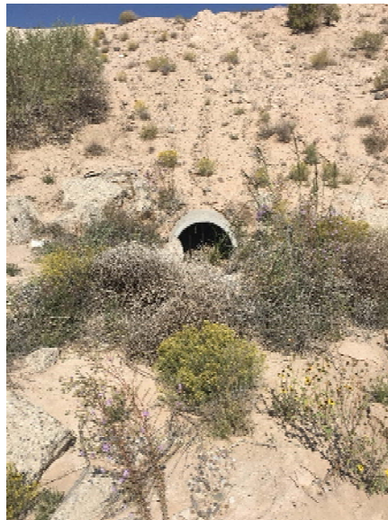
Photograph 10: Outfall 35B is a grated concrete culvert. Debris caught at the bottom of the culvert. Tumble weeds surround the culvert. No non-stormwater discharges were present at the outfall.
