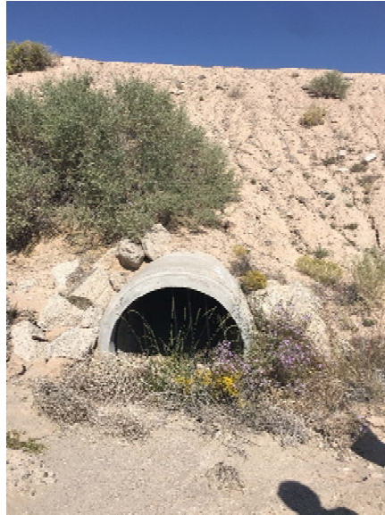
Photograph 9: Outfall 35A is a grated concrete culvert. It was observed to be dry with debris and sediment buildup.
