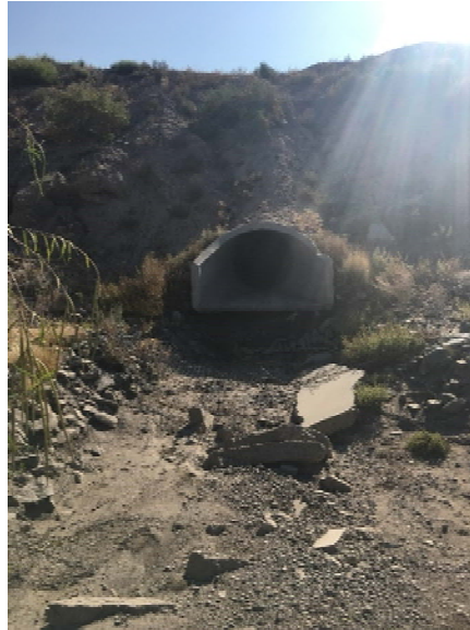
Photograph 3: Outfall 08W is a concrete culvert with metal grate. It was observed to be dry.
