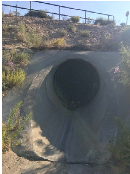
Photograph 2: Outfall SP2, a concrete culvert with metal grate, was observed to be dry. Minor trash was caught in the grate.
