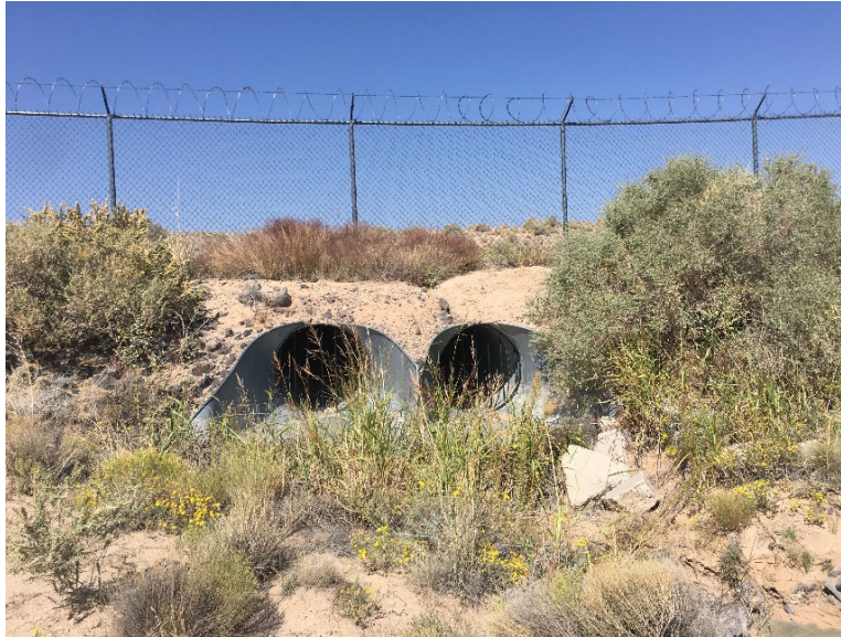
Photograph 7: Outfalls S35A and S35B are twin metal culverts with grates. Outfalls were observed to be dry.
