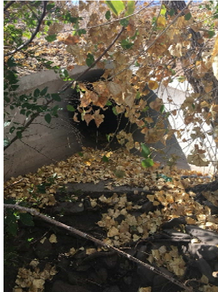
Photograph 5: Outfall CRNW is a concrete outfall (no grate). It was observed to be dry. Leaves and some litter were observed.
