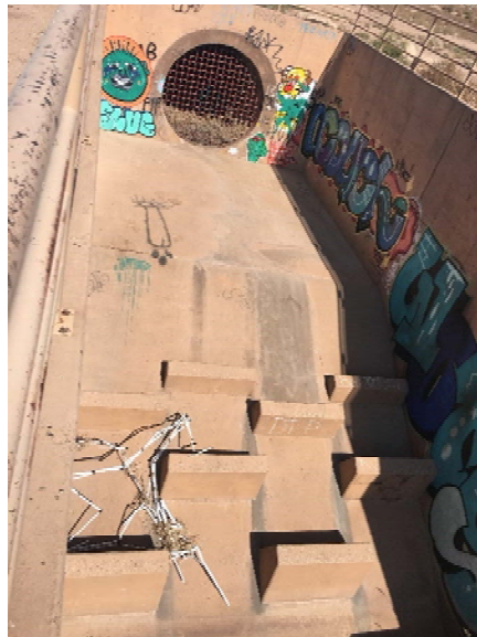
Photograph 6: Outfall W3S. No flow or standing water observed. Minor debris caught in grate. Trash in the energy dissipation structure.
