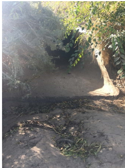
Photograph 4: Outfall CRNE is a concrete culvert (no grate). It was observed to be dry.
