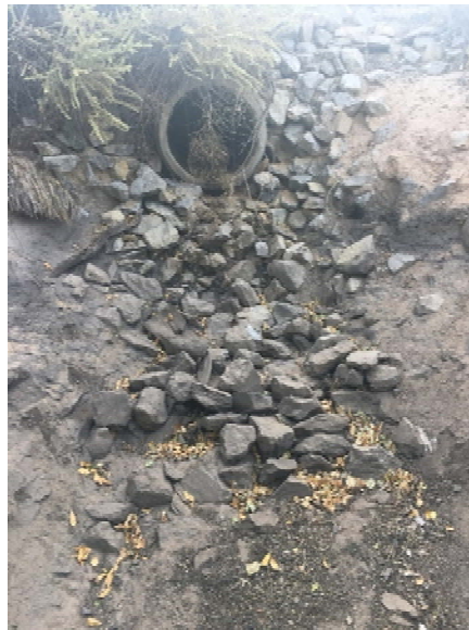
Photograph 1: Outfall SP1, a concrete culvert with metal grate was observed to be dry. Minor debris was caught in the grate.
