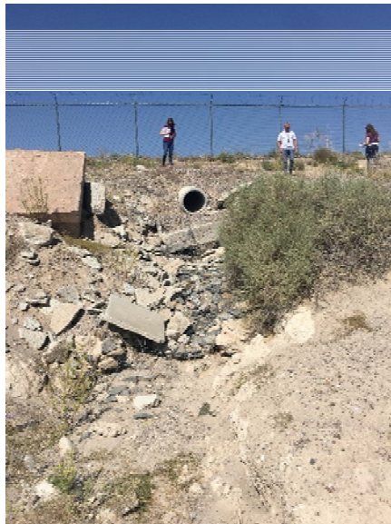
Photograph 12: Outfall W3W is a concrete culvert. It was observed to be dry and in good condition
