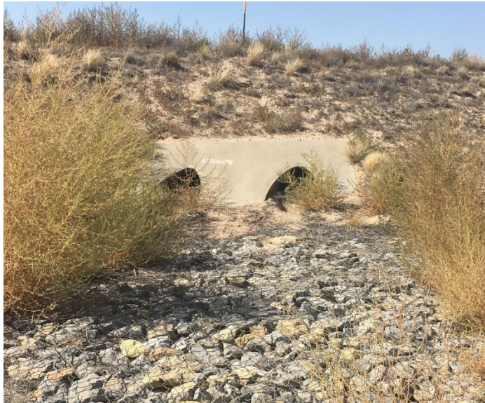
Photograph 8: Outfall 00H is a double concrete culvert. Moderate sedimentation and tumbleweed accumulation. Dry, no flow.
