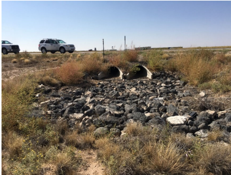
Photograph 5: Outfall 00E is a double concrete culvert. Minor tumbleweed accumulation. Dry, no flow.
