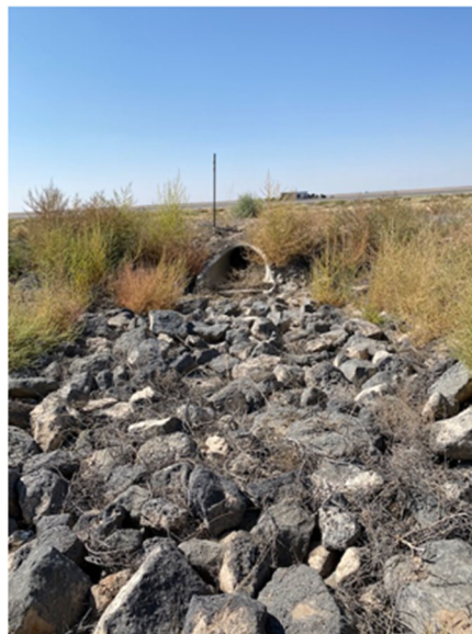
Photograph 2: Outfall 00B is a single concrete culvert. Tumbleweed accumulation was moderate. Outfall was observed to be dry.
