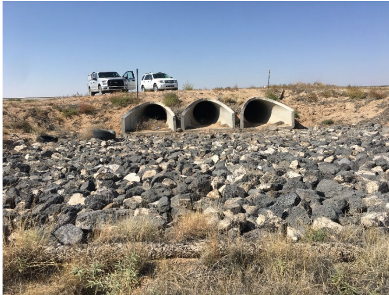
Photograph 1: Outfall 00A is triple concrete culvert. No flow was observed. Minor tumbleweed accumulation.
