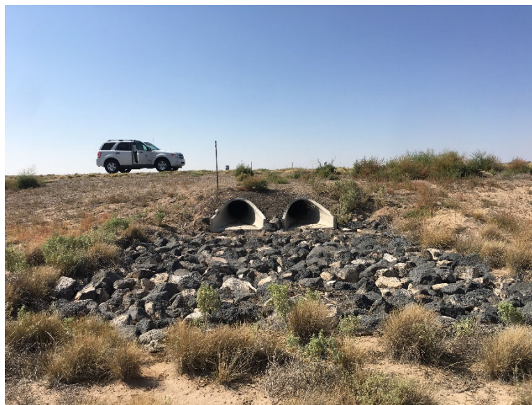
Photograph 4: Outfall 00D is a double concrete culvert. Minor tumbleweed accumulation. Dry, no flow.
