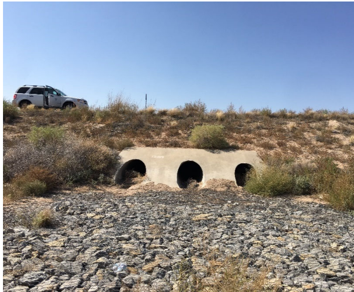
Photograph 7: Outfall 00G is a triple concrete culvert. Moderate tumbleweed accumulation. Dry, no flow.
