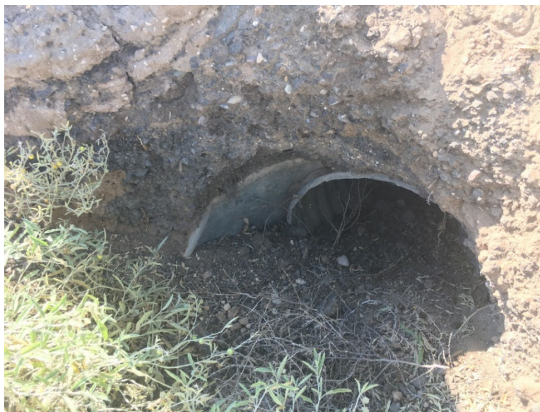
Photograph 10 Close-up view of Outfall 001. Significant sedimentation accumulation. Dry, no flow.
