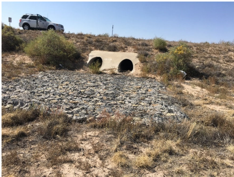
Photograph 6: Outfall 00F is a double concrete culvert. Moderate tumbleweed accumulation. Dry, no flow.
