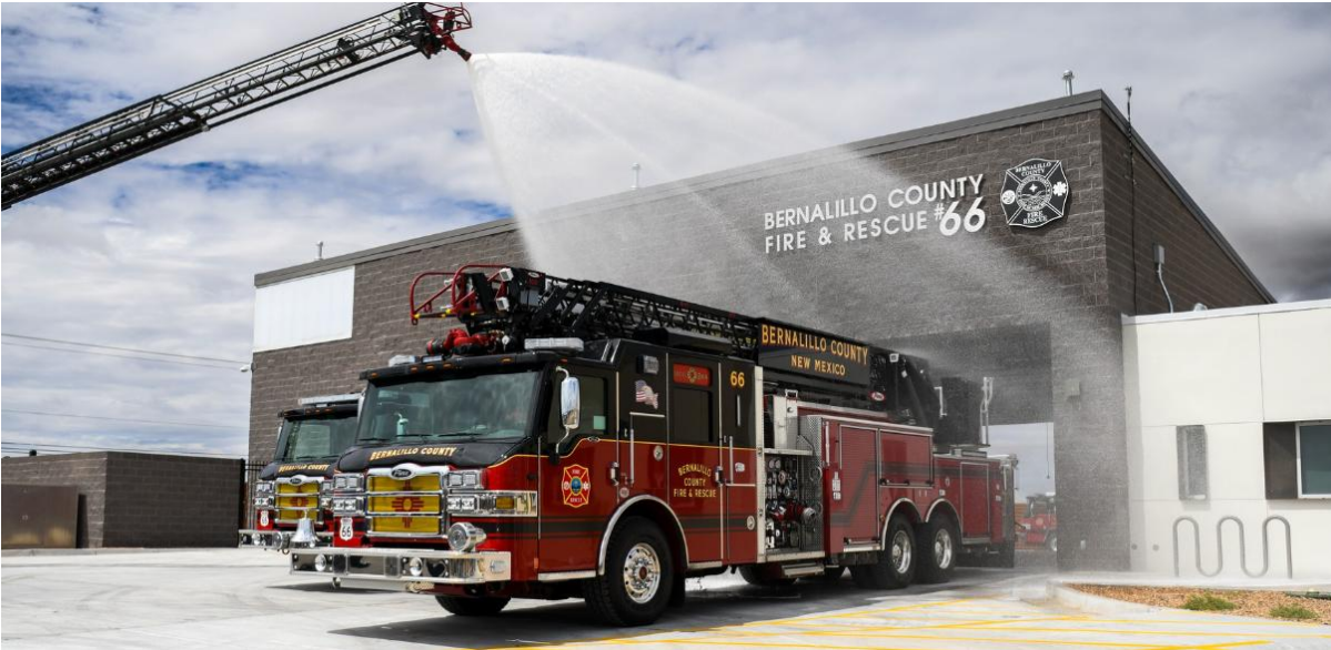
Figure 3-11. Bernalillo County Fire Station #66
